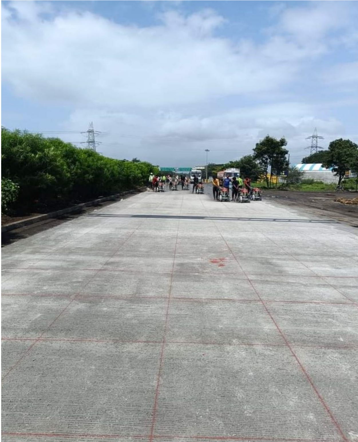
Joint Marking Work In progress
