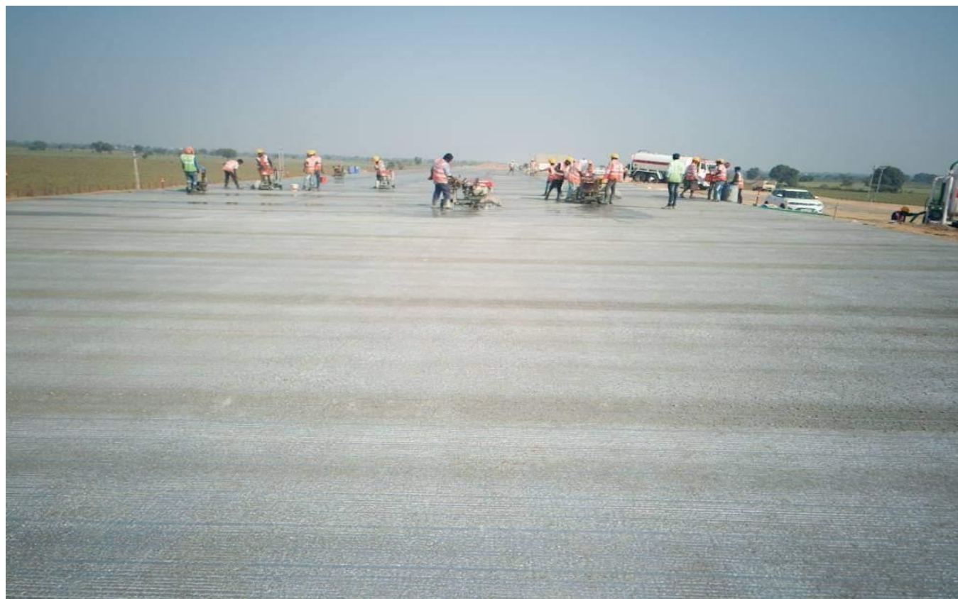
PQC JOINT CUTTING IN PROGRESS
