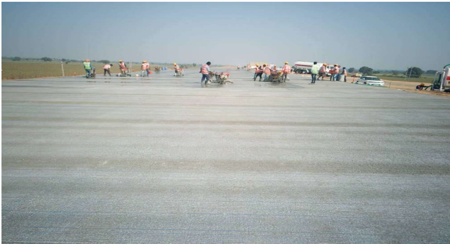
PQC Joint Cutting .
