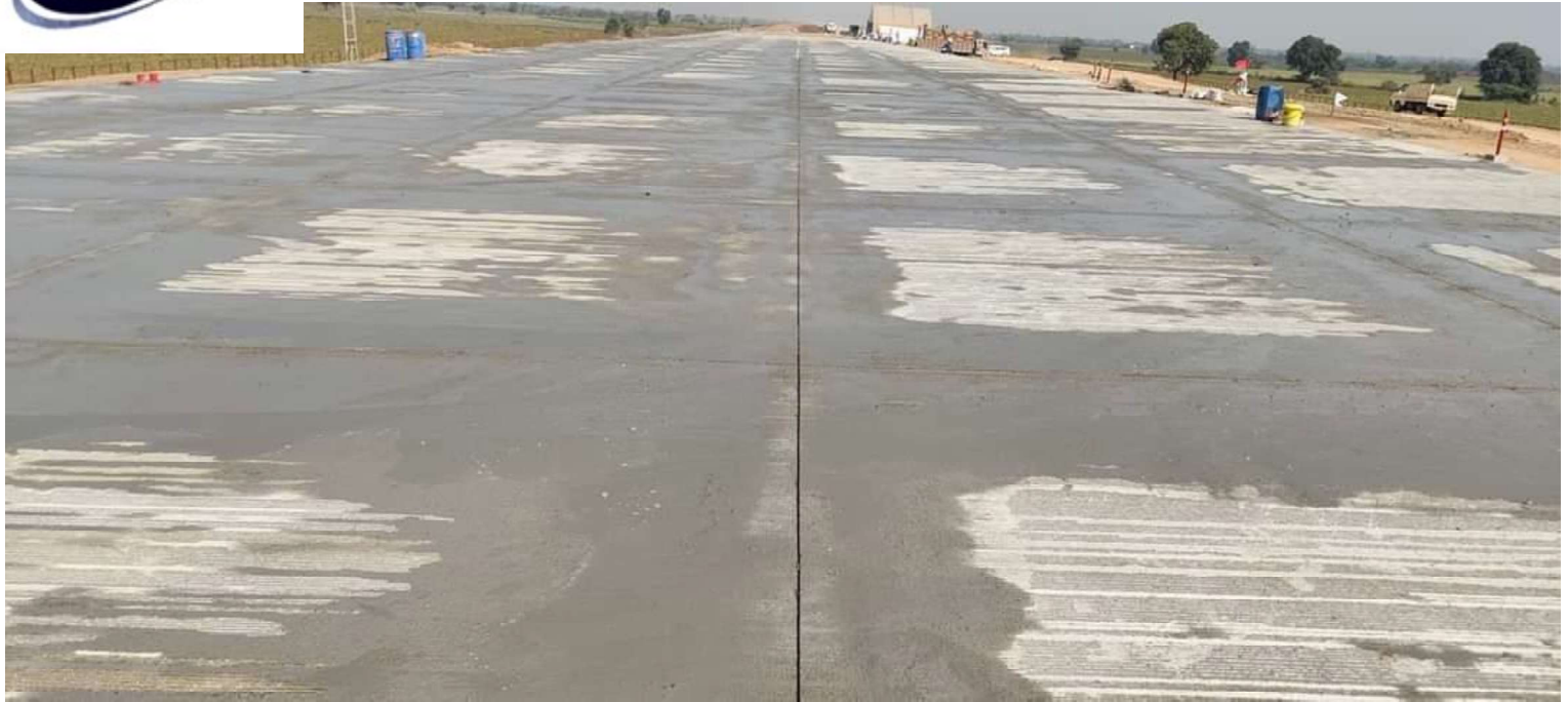
After Joint Cutting Site Photo.
