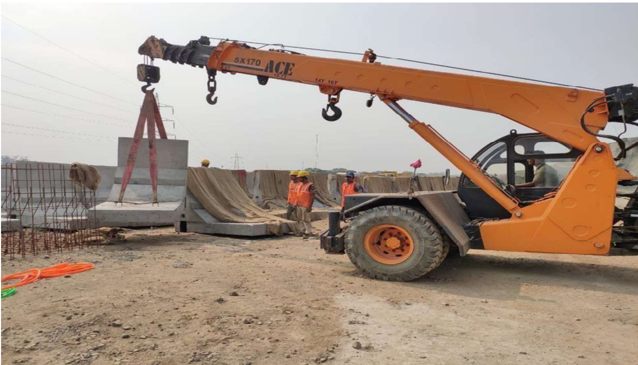
Friction slab with crash barrier Precasting
