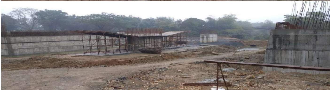
MJB AND RCC GIRDER WORK IN PROGRESS
