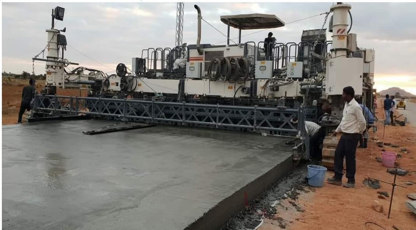
PQC LAYING WORK IN PROGRESS
